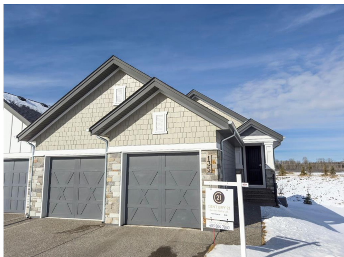
135 Clear Creek Pl, Rural Rocky View County, AB
